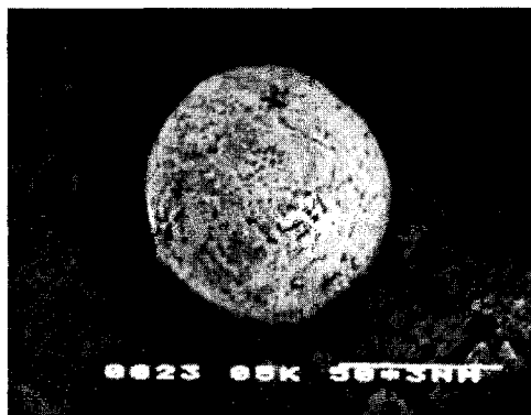
FIG. 15. Pore in Concrete
