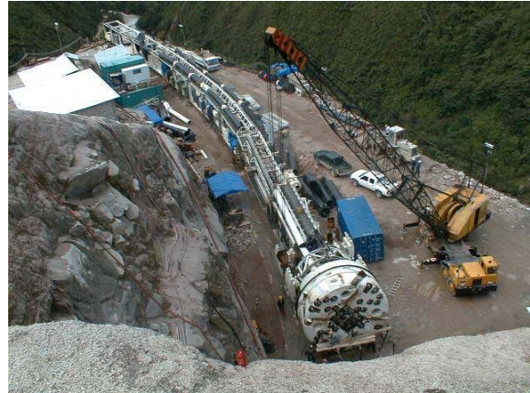
Figure 13: A typical hard rock tunnel boring machine (TBM)
